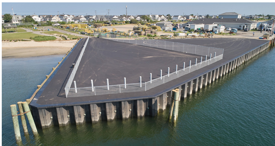
Reconstructed Seabrook Seawall in Seabrook, NH. Photography by Derrick Feole Images.
